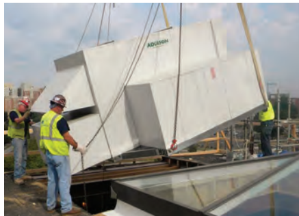
Warm in the winter, cool during summer. Contractors with Forrester Construction installed, with the utmost of care, a heating and air conditioning system in the historic Gales School.
