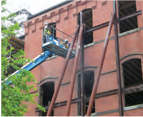
Celebrating a renovation milestone: workers remove the supporting braces from the Gales School newly reinforced exterior.
