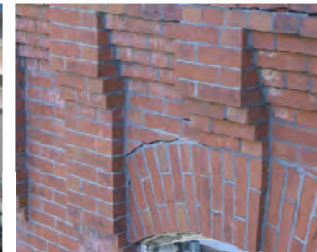
Window Head Corbelling Detail
